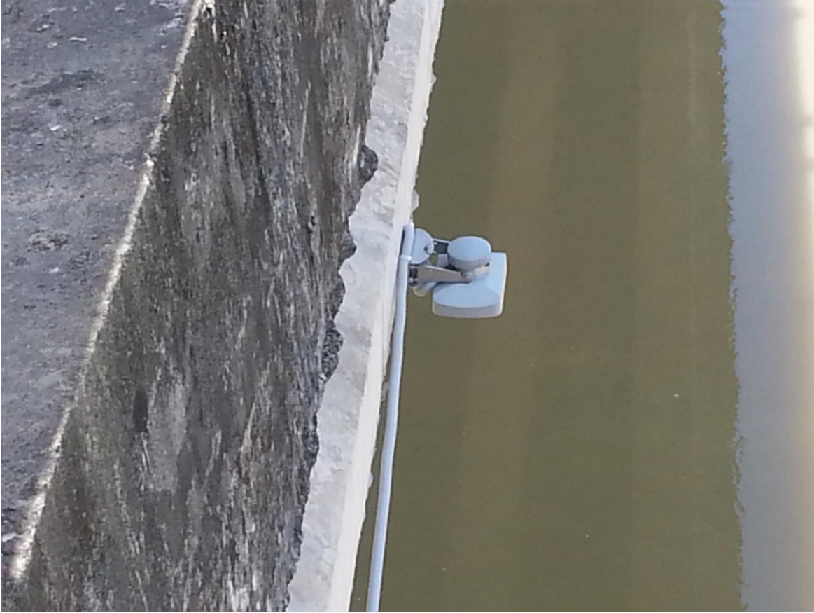
Figure 14: Radar Level Sensor mounted on a bridge
