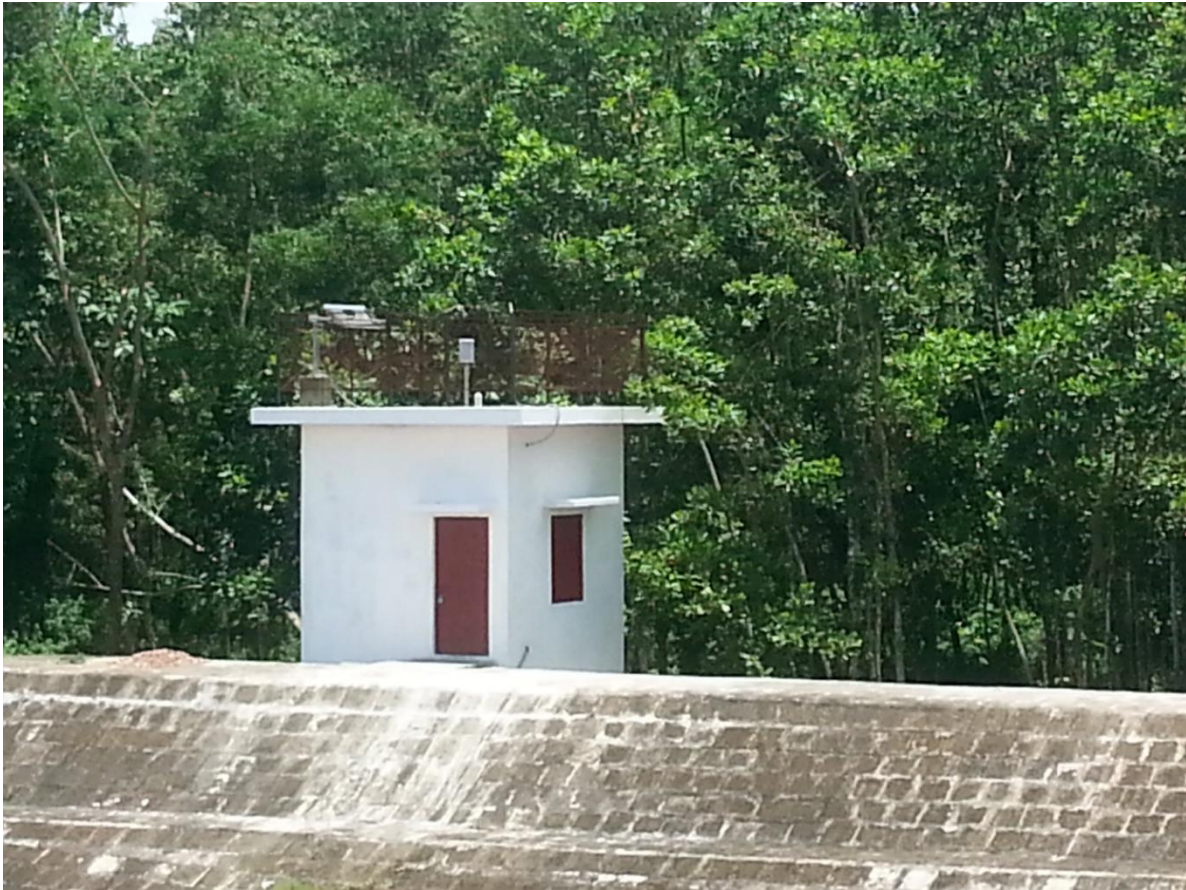
Figure 16: Tipping Bucket and Solar panel roof mounted on top of gauge house
