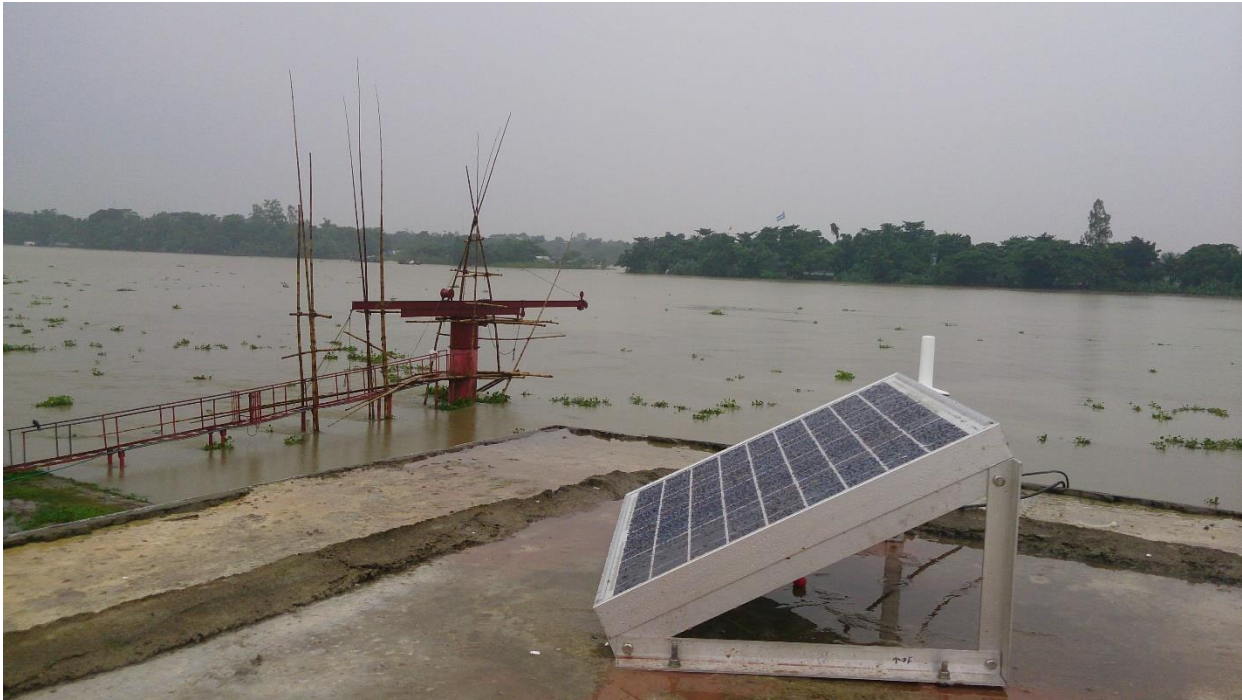
Figure 12: Solar Panel roof mounted on top of gauge house
