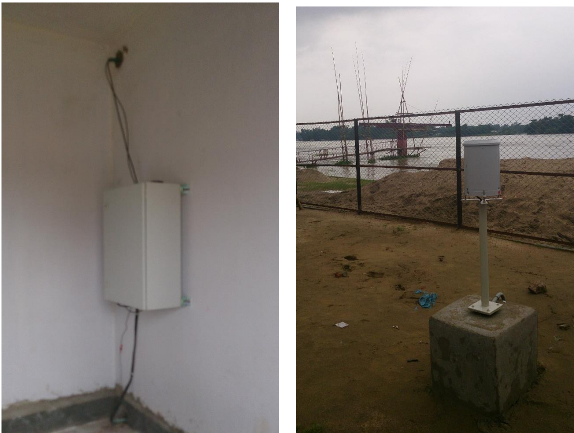
Figure 11: DCP Box wall mounted inside the gauge house and the tipping bucket
