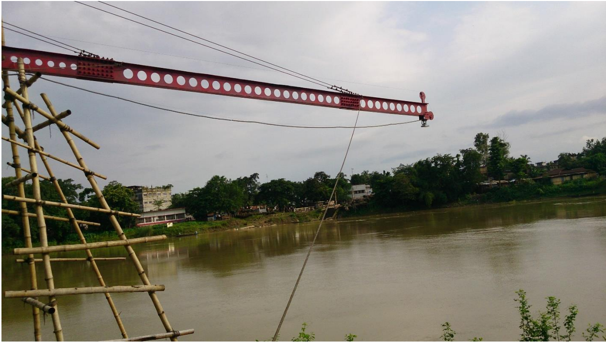
Figure 8: Metal Structure for Radar Level Sensor
