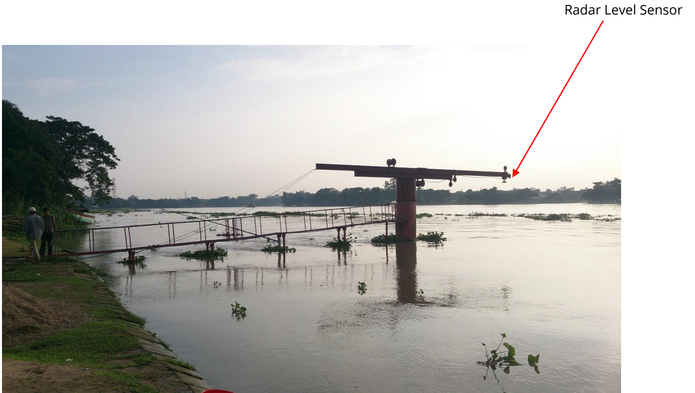
Figure 10: Metal Structure for mounting radar level sensor
